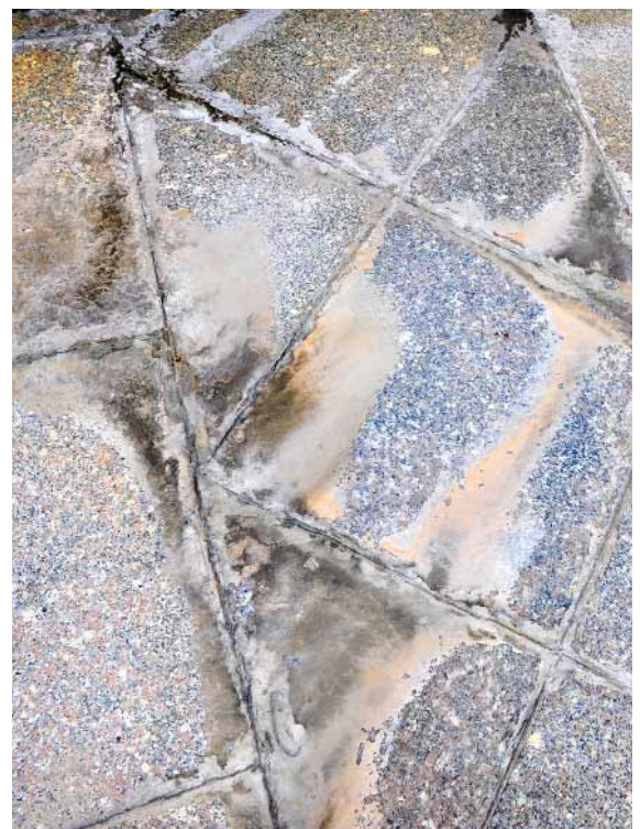
Unsightly efflorescence
